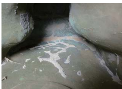
Figure 39. Sand residues detected inside the work.
